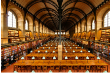
Metal covering of the reading hall of Sainte-Geneviève library by Labrouste, opened in 1851.
