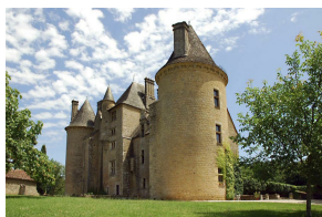
Chateau of Montal restored by Maurice Fenaille.
