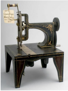
Sewing machine by Isaac Singer, patented model from 1851 and presented at the 1855 World's Fair. National Museum of American History, Washington.
